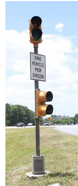
Figure 5: Ramp Meter Signal Assembly Example
