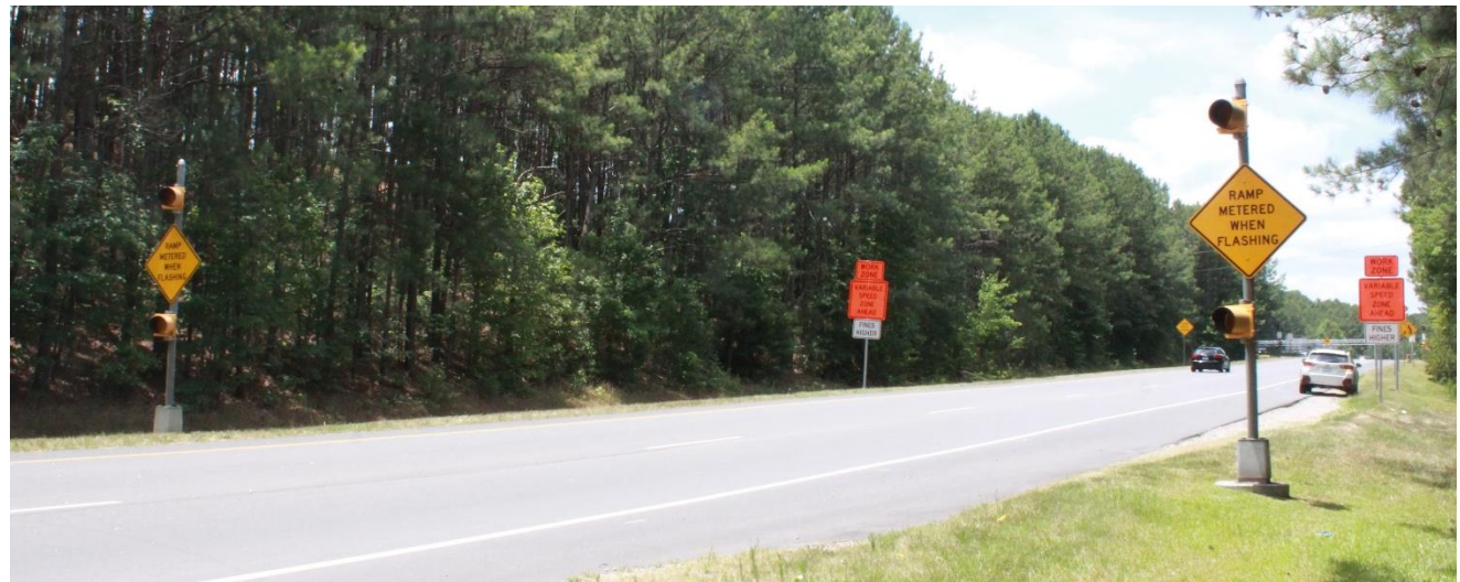
Figure 4: Advance Warning Beacon Assembly Example
