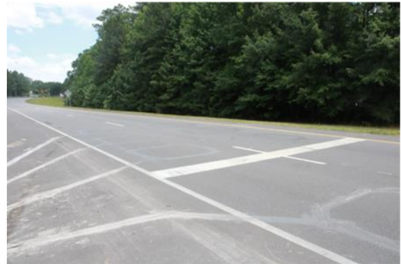
Figure 8: Passage and Demand Detection with Induction Loops
